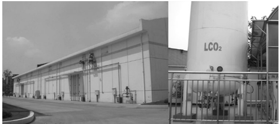
Fig. 7 Application of CO 2 based CA on a 5,000 tonnes concrete horizontal silo bin and the CO 2 gas supply from the tank in Mianyang, Sichuan, China
