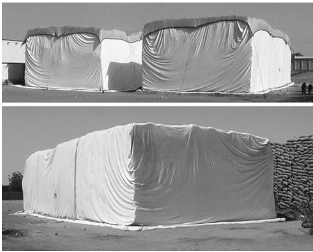
Fig. 10 Hermetic storage of cereals in 1,050 tonnes MegaCocoon™, Sudan
