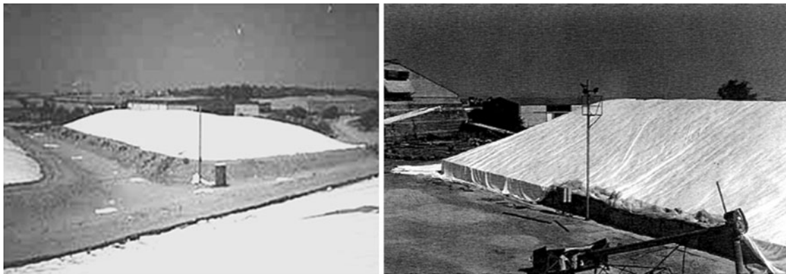
Fig. 8 Bunker storage for conservation of large bulks of 10,000–15,000 tonnes capacity (Navarro et al. 1984, 1993)
